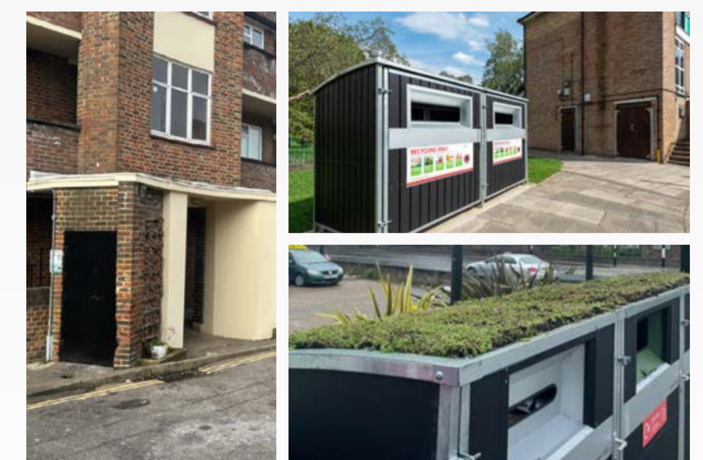
Existing bin stores connected to internal chutes
