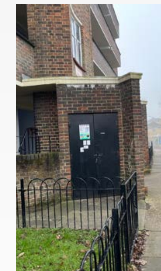
Existing bin stores connected to internal chutes
