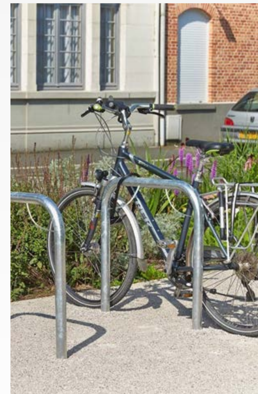
Example of 'Sheffield' cycle stands for visitor parking that could be provided
