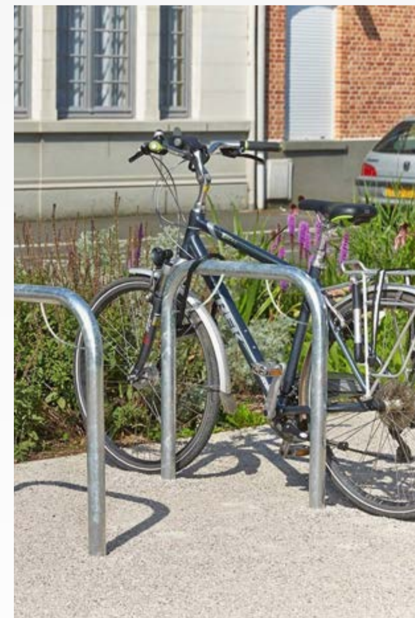
Example of 'Sheffield' cycle stands for visitor parking that could be provided
